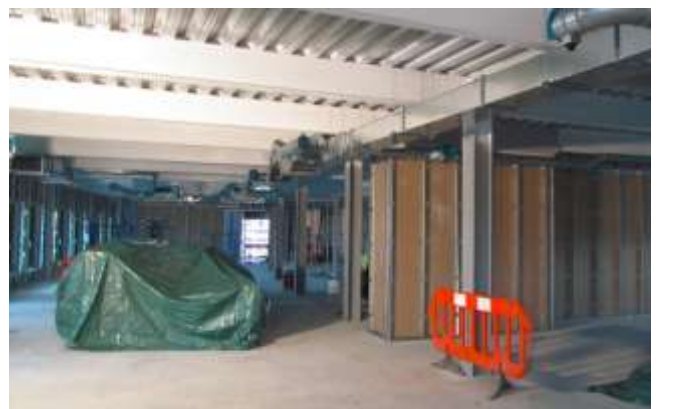
Construction Progress Photos
