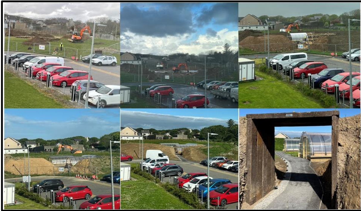
Figure 3.6: Polytunnel build progress from April 2022 to start of July 2022.
